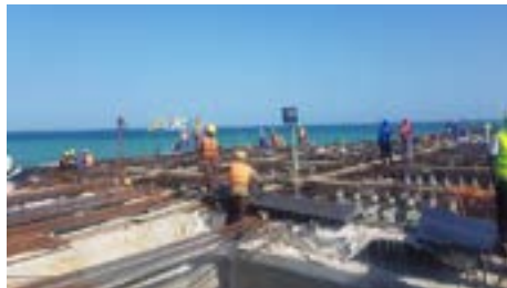
Lamu Port Berth!! Work in progress.
